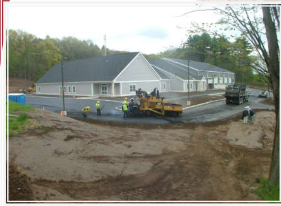
Granby Police and Fire Station, Granby, Massachusetts
